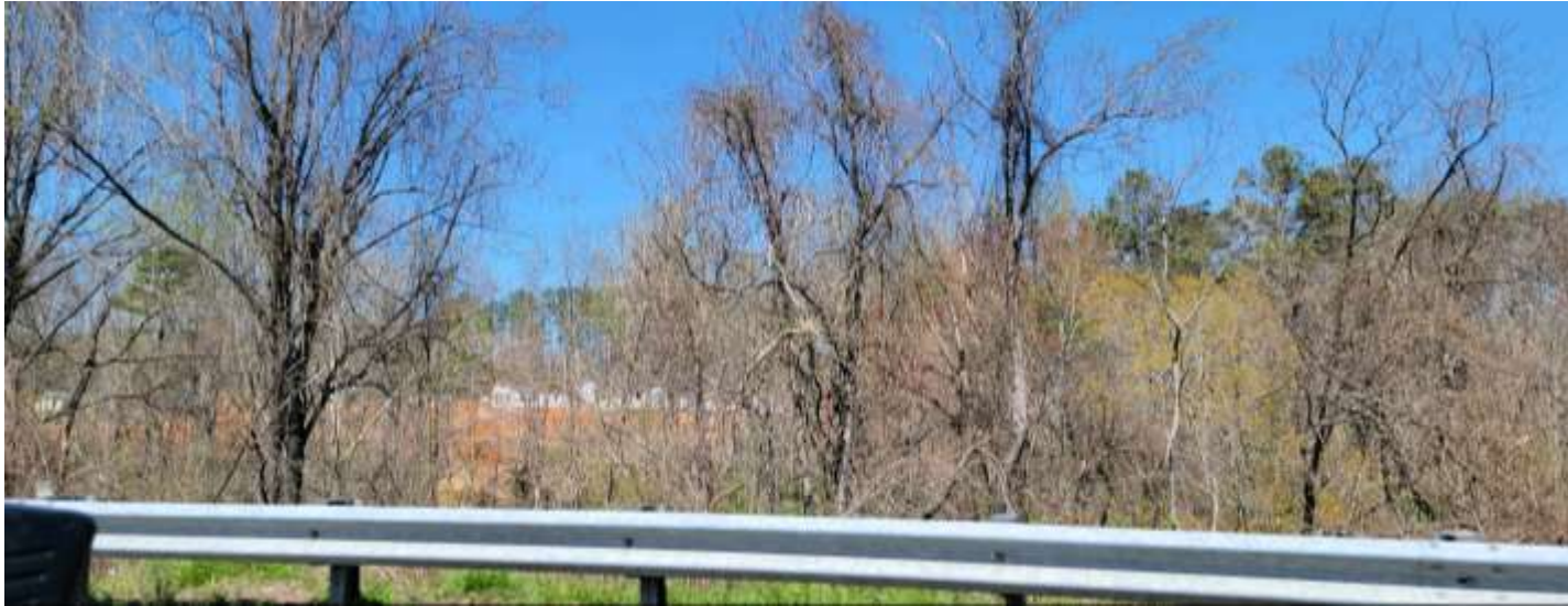
Figure 2a: View of a portion of the cleared/graded site with buildings under construction in early Spring.
